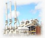
Low-cost Refining in Sao Luis
