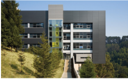
Designed with Kawneer Curtain wall and LEED Gold-certified, the Lawrence Berkeley National Lab building consumes 28% less energy than the already rigorous California building efficiency standards. The sustainable, energy efficient building maximizes daylight, and its project-out windows increase occupant comfort by helping improve air circulation and natural ventilation.
