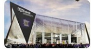
Arconic's Kawneer curtain wall and entrances of the Minnesota Vikings stadium
